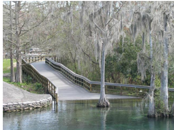
New Access Ramp at Blue Run of Dunnellon Park
