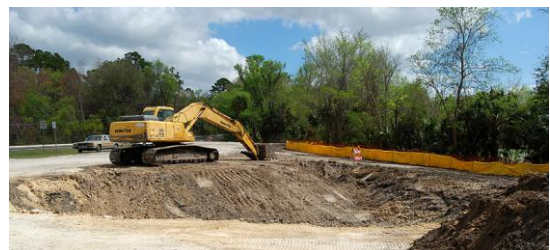
Blue Run Park stormwater improvement construction
