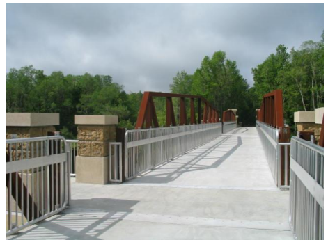
New trail bridge across Withlacoochee River
