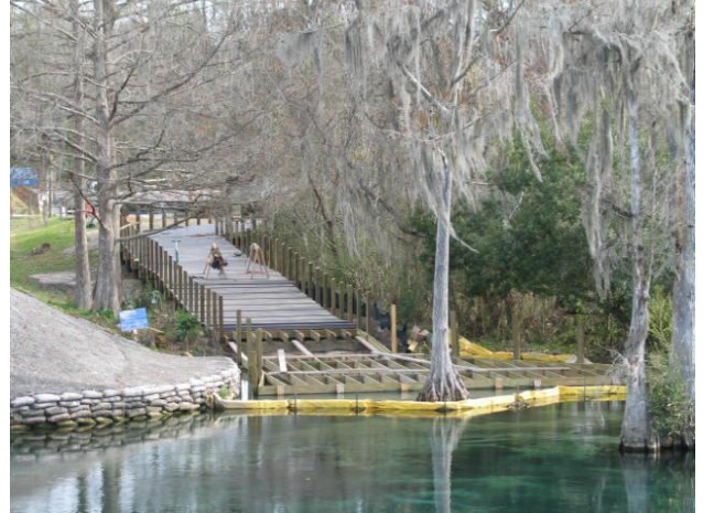
Progress on river access ramp at Blue Run of Dunnellon Park
